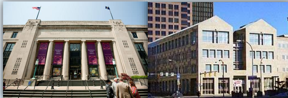
Central Library of Rochester South Avenue
